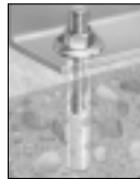
Doweling into Concrete with Rebar
